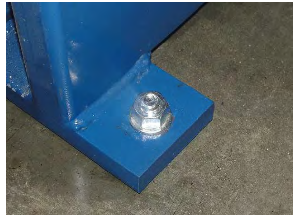
Anchor Bolts in position.
